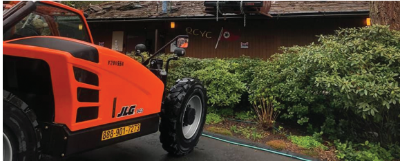
Outstation roof replacement underway - photo by Bob Schrader
