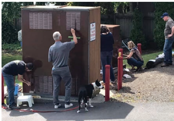
Outstation orientation crew painting transformer boxes
