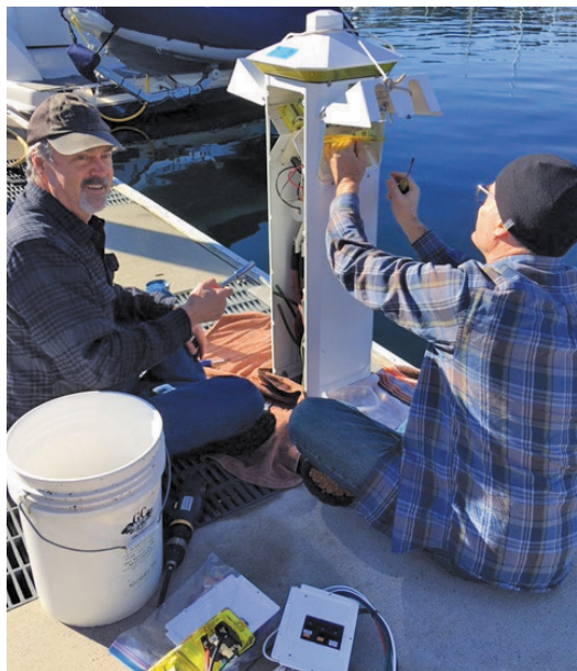
VESC volunteer crew Duane Engle and Tim Hicks replacing outlets
