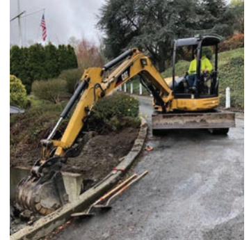
Excavator called to find broken water main from street
