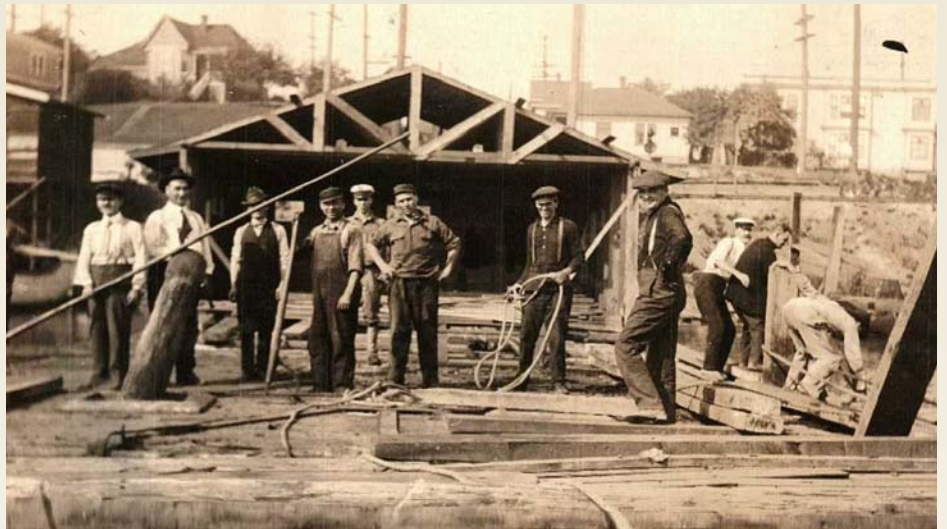
Volunteers put logs under an 'old scow' to create the floating clubhouse
